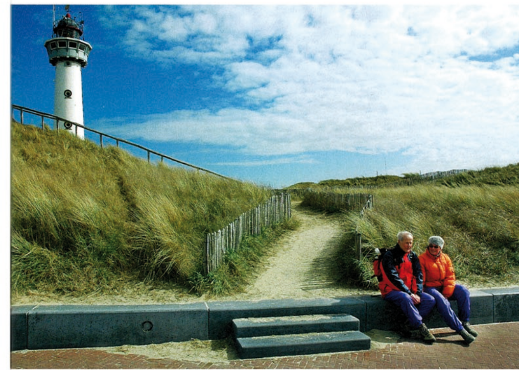
The plinth along the circular dune on which the Jan van Speyk lighthouse stands.
