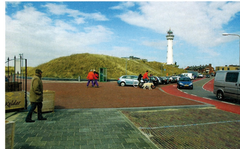
The renovated walk around the lighthouse. The pavement in front is not renovated yet.
