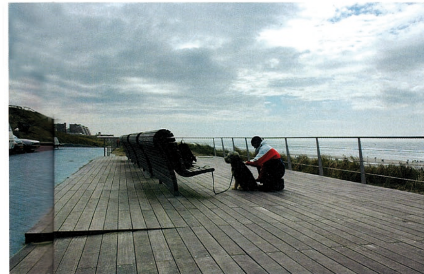
Wooden dune balconies with eye-catching benches.
